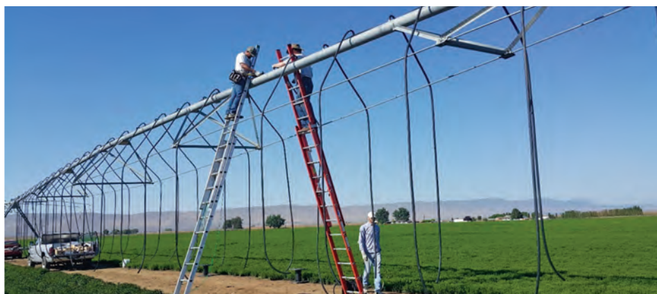
Fig. 1. Converting three spans of center pivot in mint field in Toppenish from MESA to LESA/LEPA.
