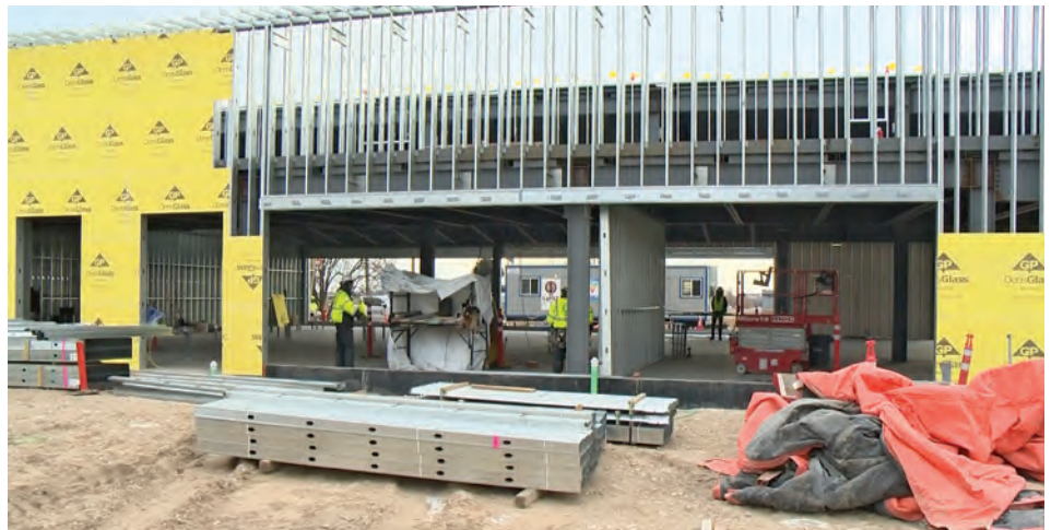
Construction of the new Idaho Center for Plant and Soil Health
